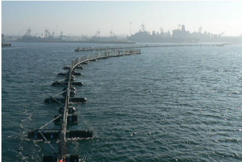
Figure 5-2 Boat Barrier System (Port Security Barrier)
