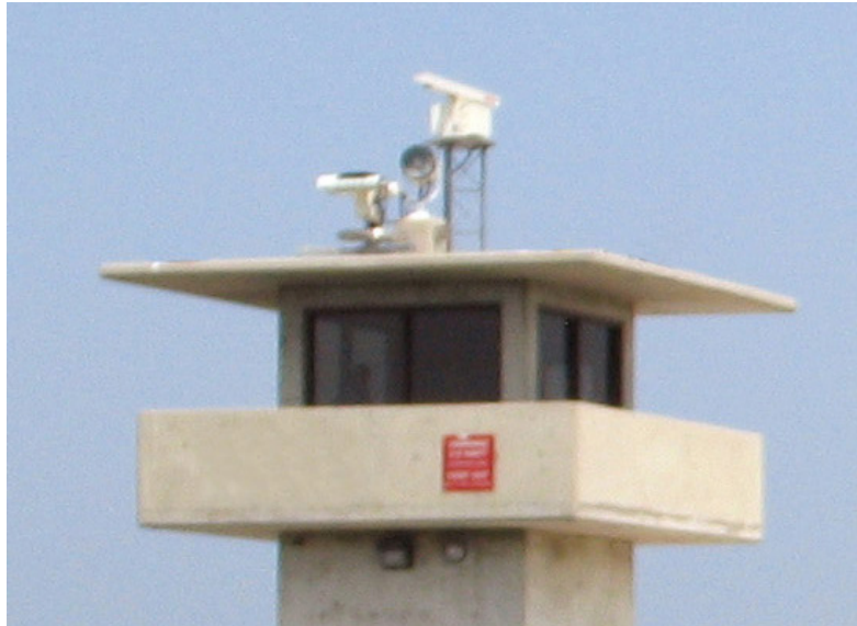
Figure 5-6 Roof Mounted Equipment
